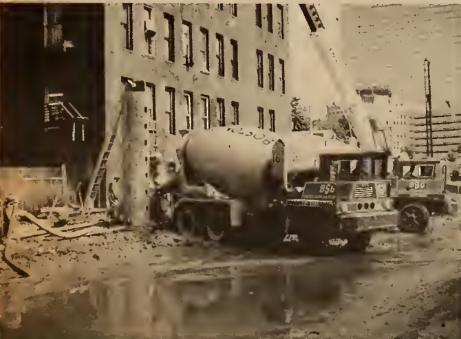
Step 4: Concrete Pouring and Slurry Removal.
